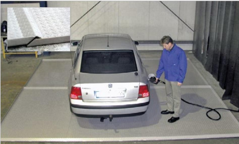
**Filling point for diesel and biodiesel operated only for own consumption, for indoor use or under cover**
