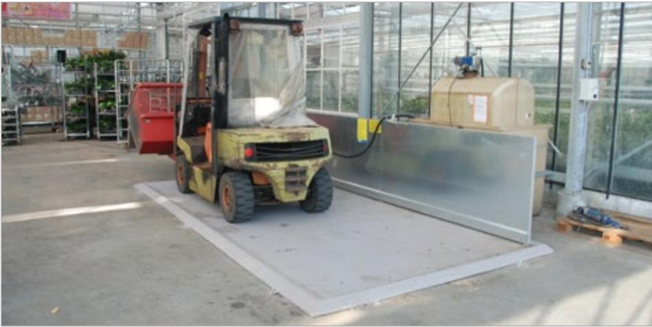
**Filling point for diesel and biodiesel operated only for own consumption, indoor use or under cover**
