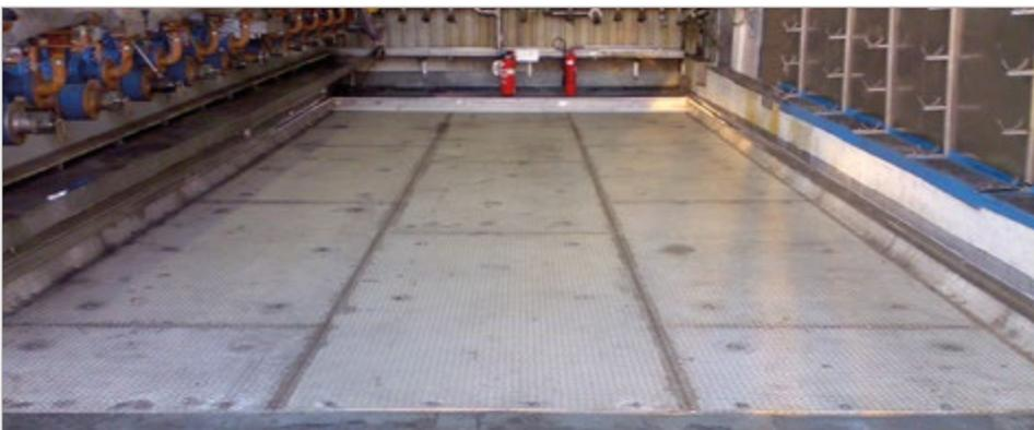
Ground protection lining made of stainless steel
