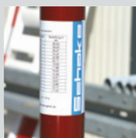
All props marked by type class and load table.
